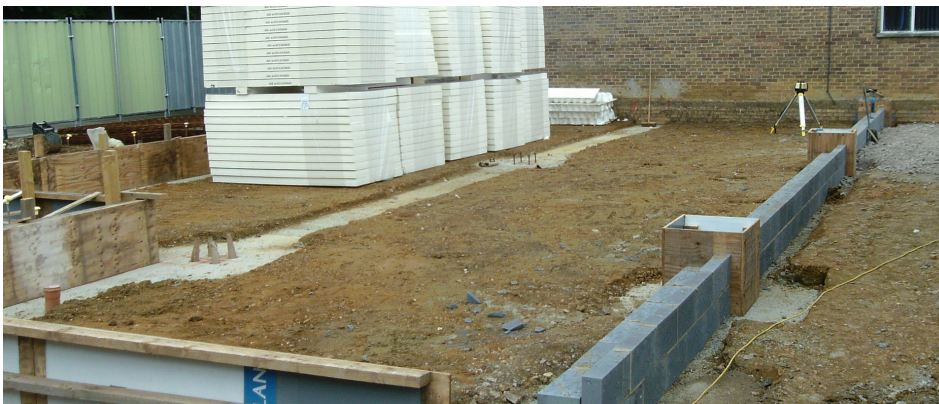
The footprint of the new building has been excavated to formation.
